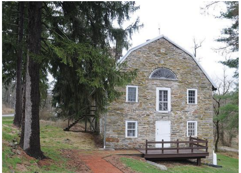
Volunteers will be renovating the historic 200-year-old grist mill at Pine Grove Furnace Park. Jason Malmont/The Sentinel
